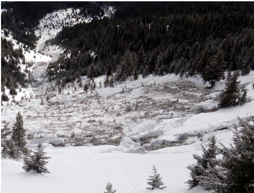
Figure 6: Looking down the Shed 11 avalanche path in John F. Stevens Canyon, Glacier National Park of a glide avalanche (GS-N-R3-D2.5-G). Photo: BNSF Avalanche Safety.
